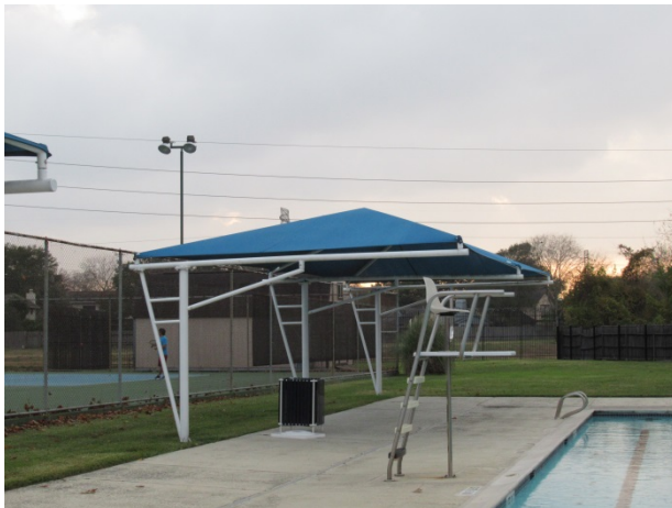
Shade structure overview
