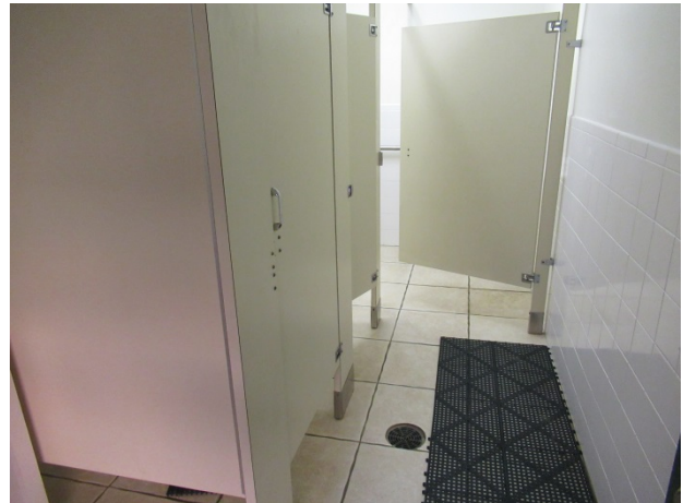
Rest room with tile wall and floor coverings
