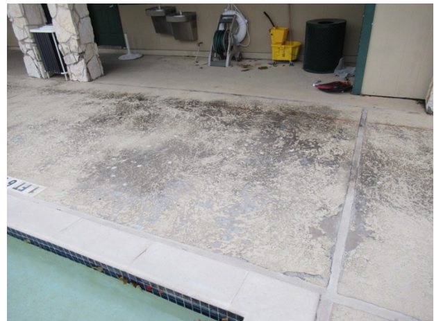
Coating deterioration
