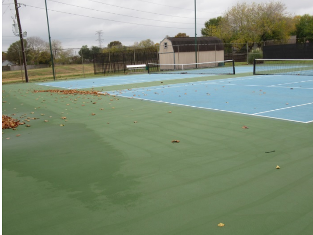
Tennis court overview
