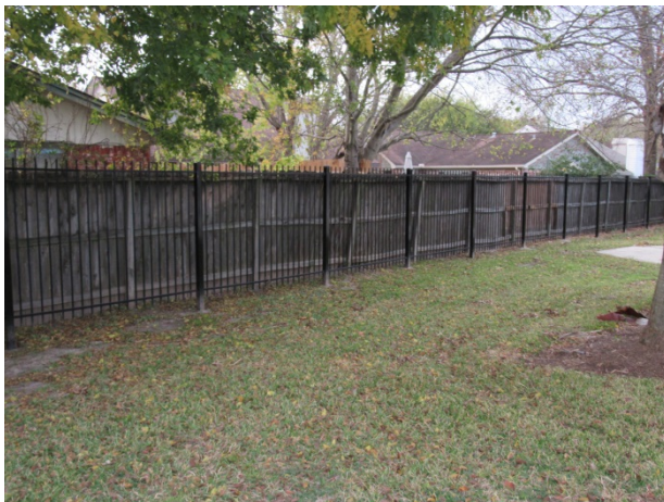
New fence overview
