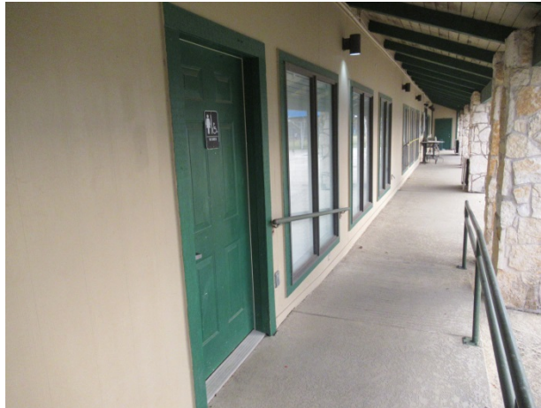
Door and windows
