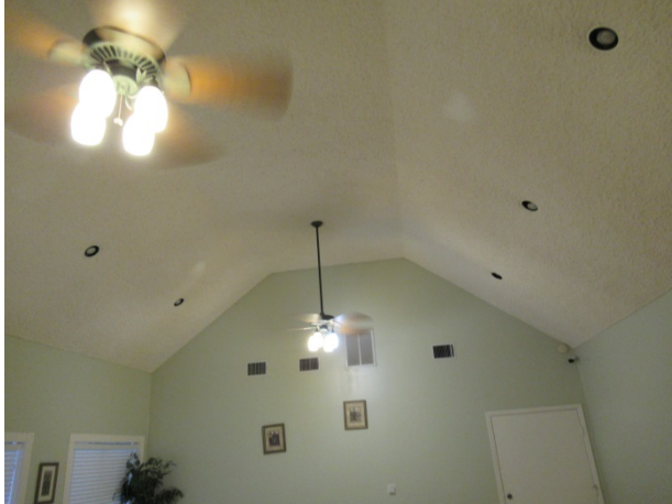
Interior paint finishes
