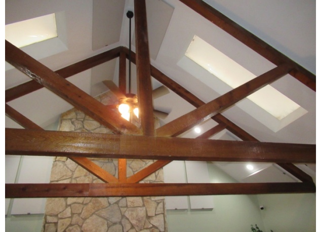
Interior paint finishes
